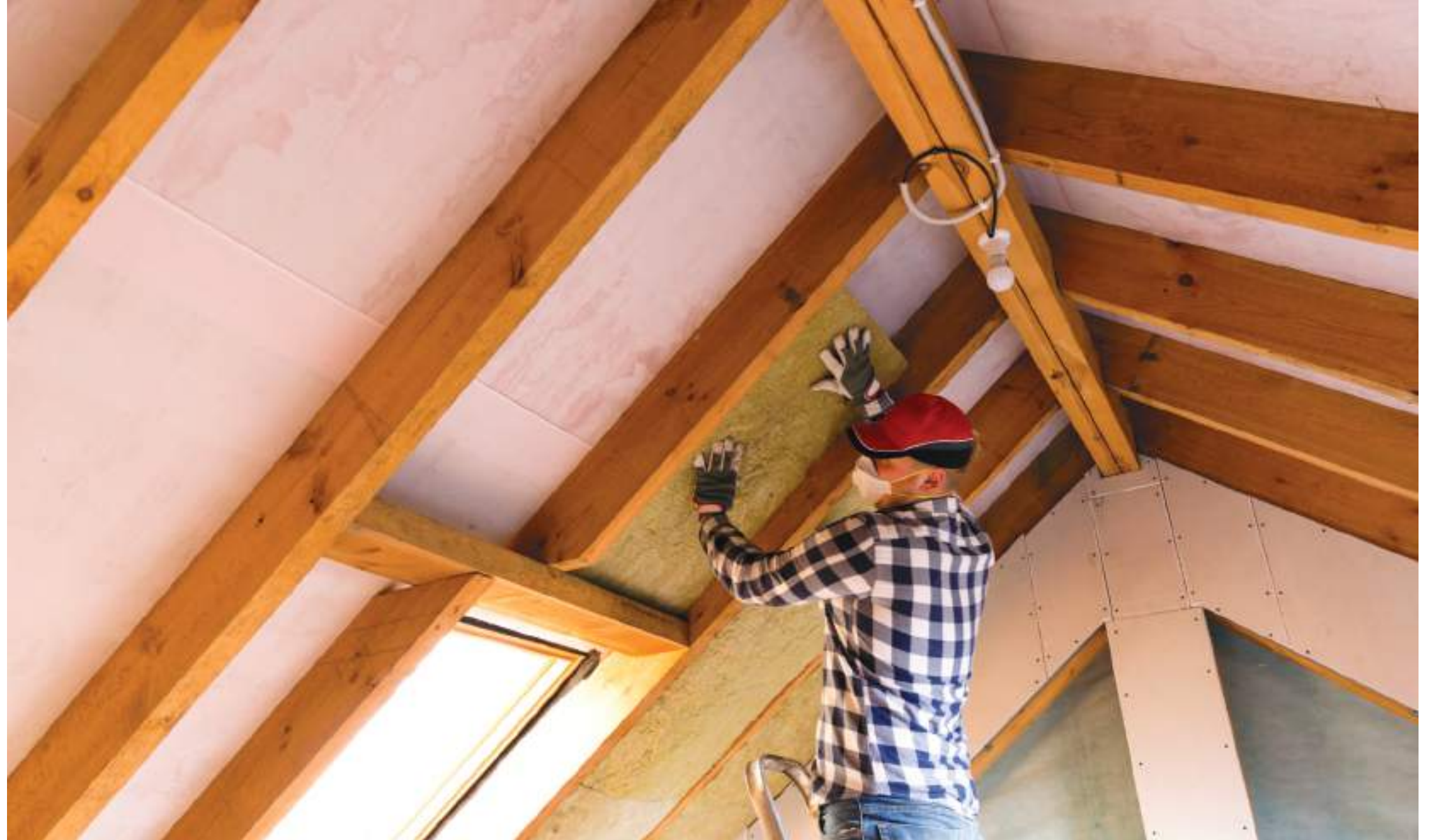
Figure 2: Installing thermal roof insulation
