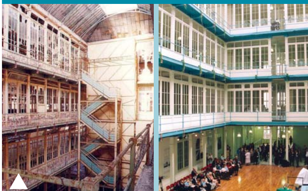
Anchor Mill interior atrium before and after restoration
