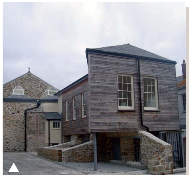
Harvey's Foundry, Hayle: After - converted to accommodate new office uses
