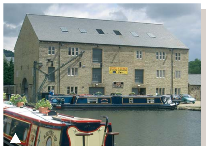
Sowerby Bridge Wharf, Warehouse No 4: After
