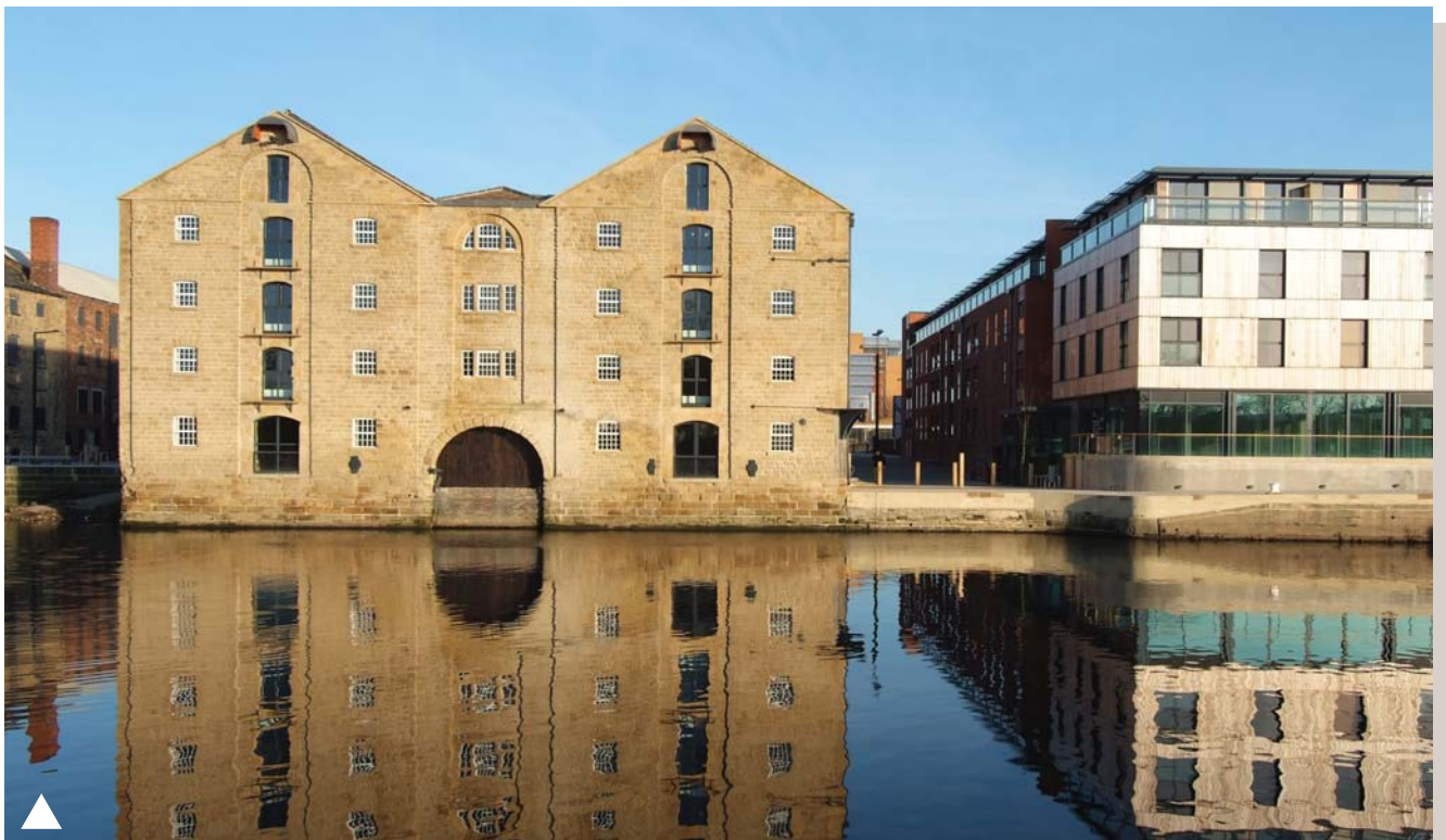
Navigation Warehouse, Wakefield: After (image courtesy of CTP St. James a Joint Venture between CTP Limited and St James Securities Limited)
