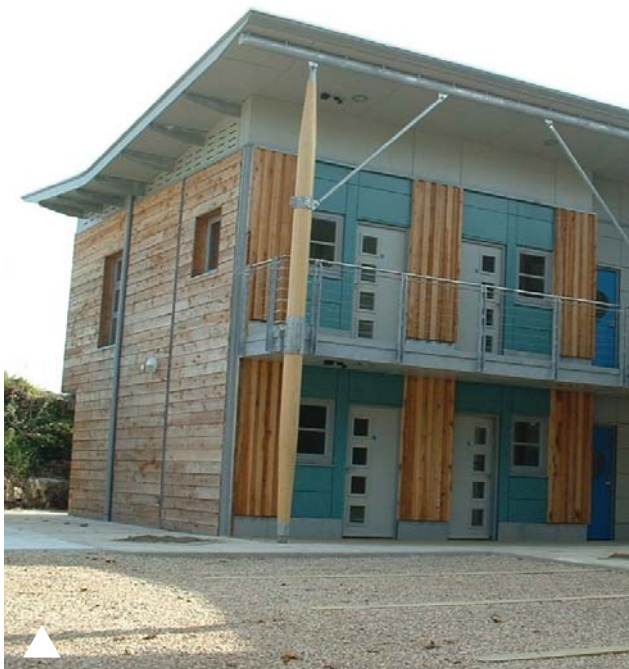
Harvey's Foundry, Hayle: Phase I. A new office building was erected using appropriate materials to a modern design. This provided space for small local businesses bringing in rental income to support the Harvey's Foundry Trust
